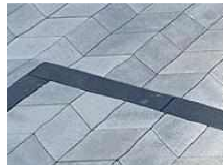
FEATURE PAVING AT LOBBY AND RETAIL ENTRANCES
